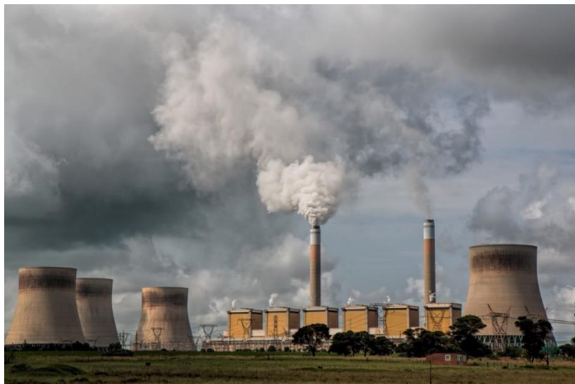
Image title: Power station
